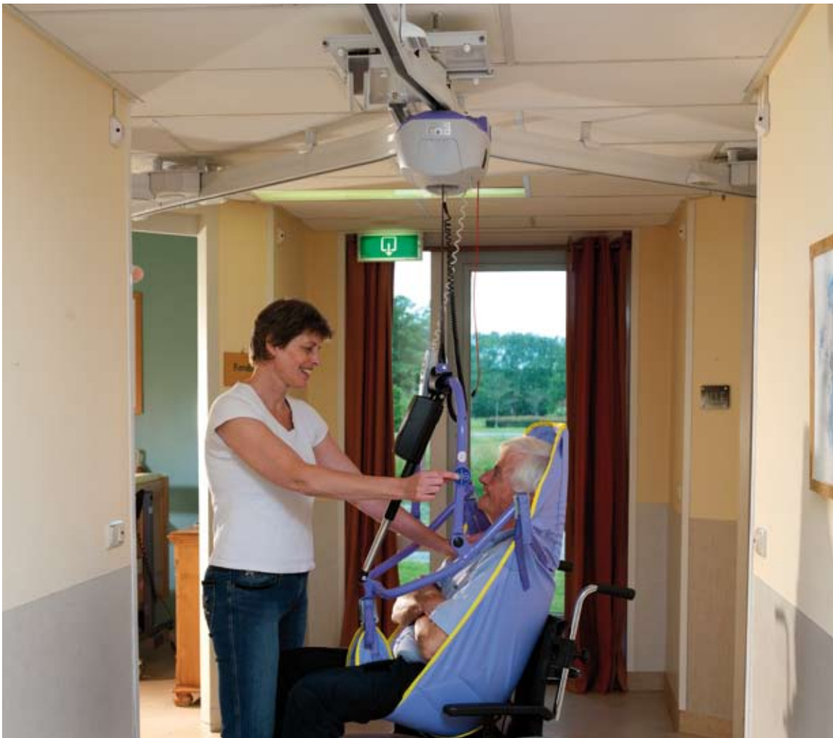
This permanent KWIKtrak solution includes an exchanger to serve two facing rooms as a shared connection to the corridor track in an elderly care facility.
