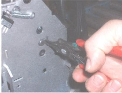
3. Remove the snap ring that maintains the strap roll shaft with the retaining ring pliers.
